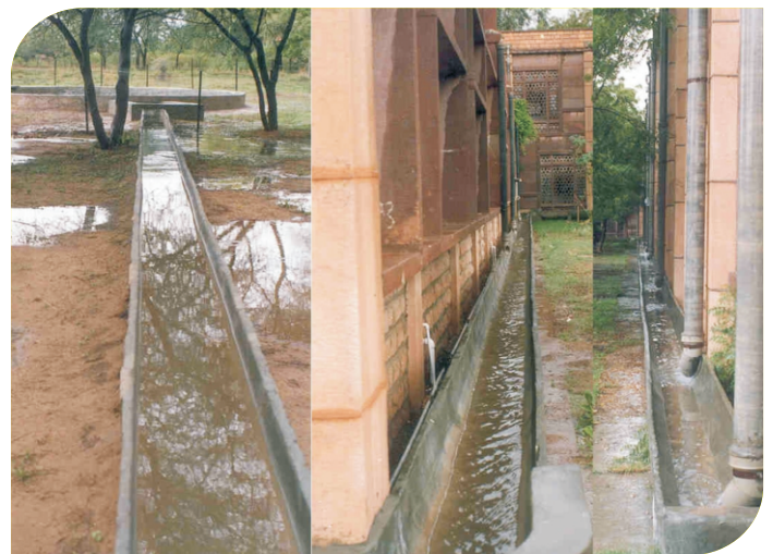
Rooftop rainwater harvesting
