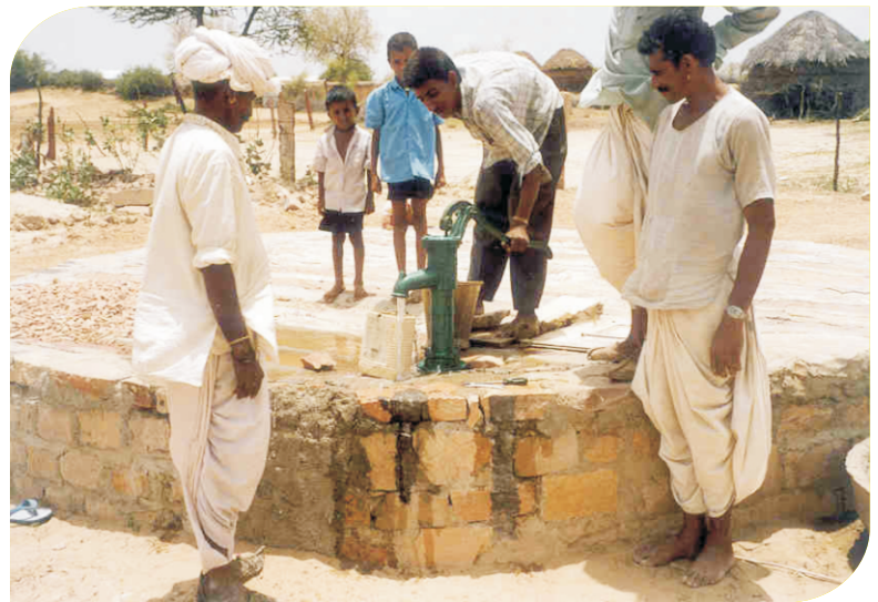
Improved tanka of 50 m 3 capacity with hand pump for safe water withdrawal
