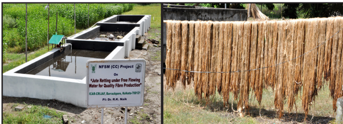
Cement tank based free flowing water system for jute retting
