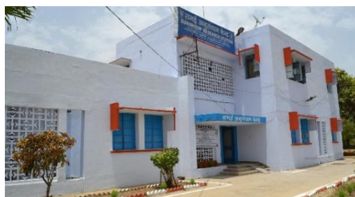
Sunnhemp Research Station, Pratapgarh
