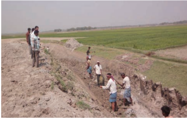
Construction of Drainage Channel in flood prone areas
