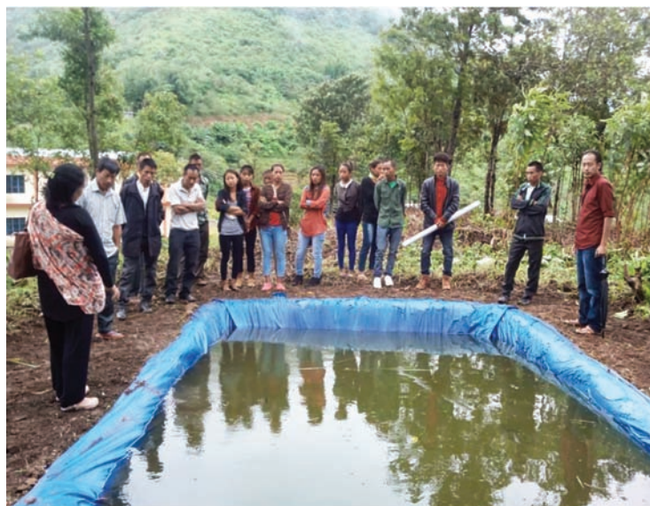
Water harvesting structure (Jalkund) in hill top of Tuensang dist.
