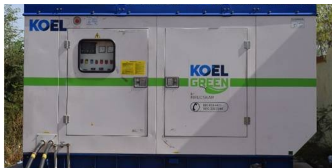
Installation of Generator (120 KVA DG)
