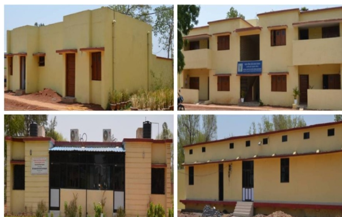
Renovated buildings of NIBSM during 2016-17
