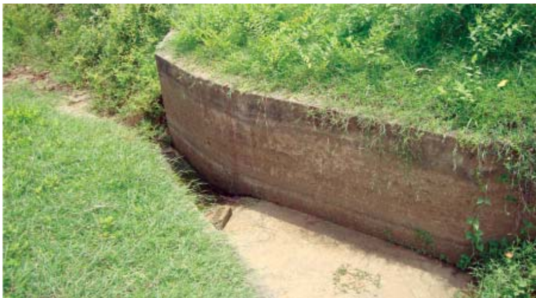
Plate 4. A flume for measurement of flow in the Atala Minor.
