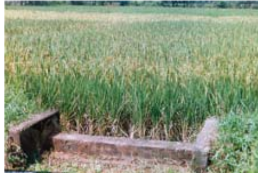
Plate 5. Experimental plot with surplus weir at the downstream side
