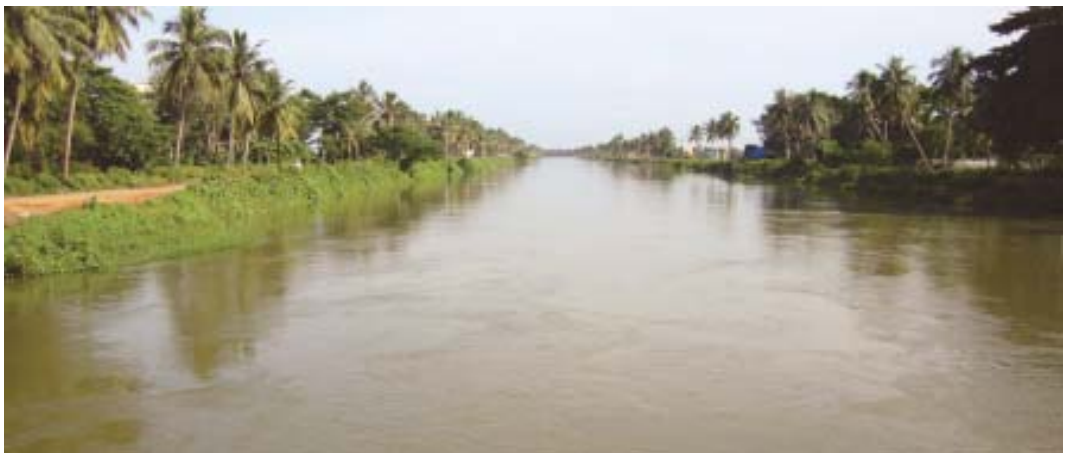
Plate 2. Puri main canal system
