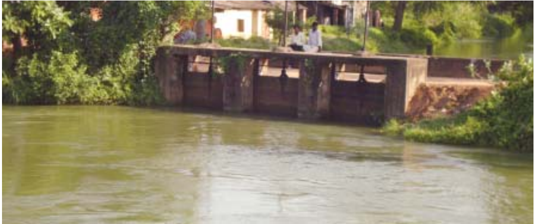
Plate 1. Head regulator of Phulnakhara distributary (off-taking from Kakatpur branch canal)
