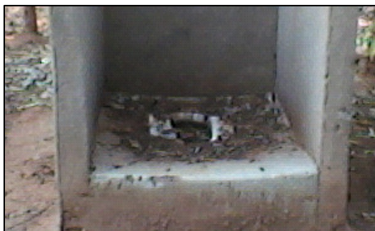
Fig. 21: TSC in bad shape in the village
