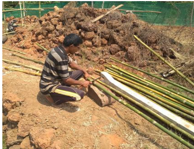
Bamboo cutting for hapa installation
