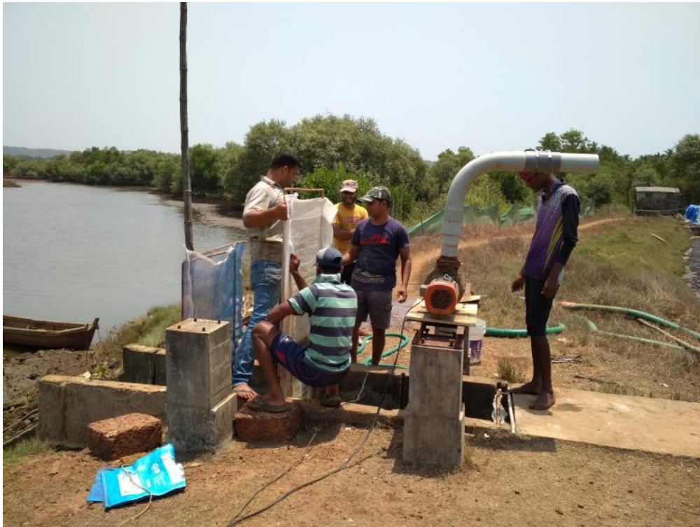
Cleaning and fixing of water screen of pond inlet system
