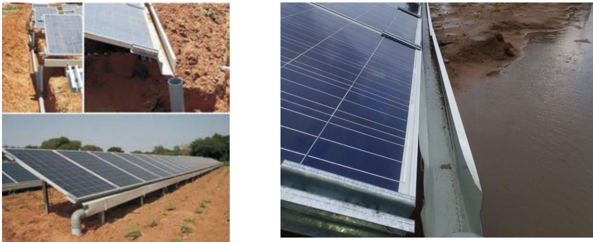
Fig. 2. Rainwater harvesting system from top surface of PV module
