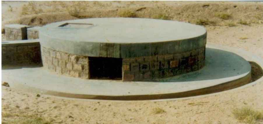
Fig. 1. Improved Tanka (21 m 3 Capacity)
