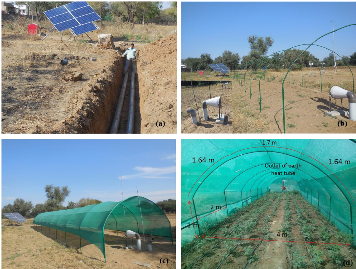
Fig. 4: Protected agriculture system with earth tube heat exchange systems with a fan motor operated by solar PV pumping system (1 hp AC pump).
