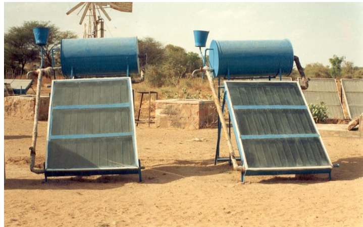
Fig. 1. Solar water heater with GS-Al and Cu-Cu collector
