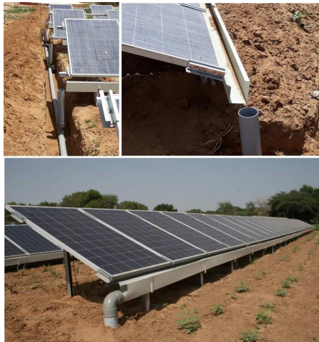
Fig. 6: Rain water harvesting system from top surface of PV module
