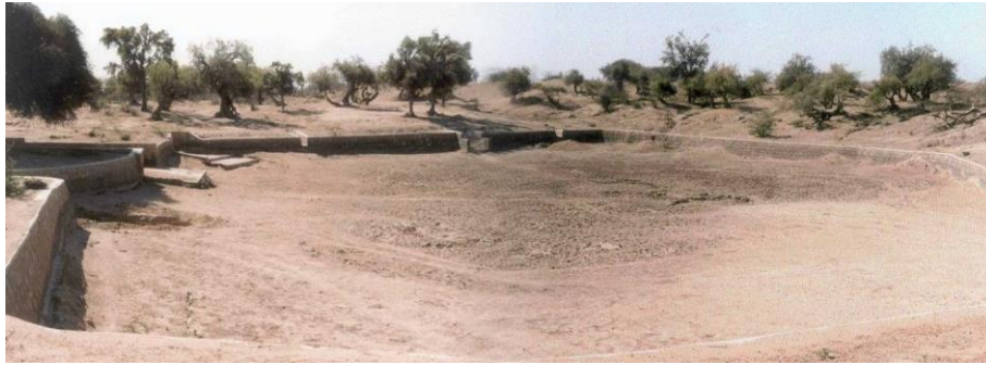
Fig. 4. Improved nadi with inlet and outlet
