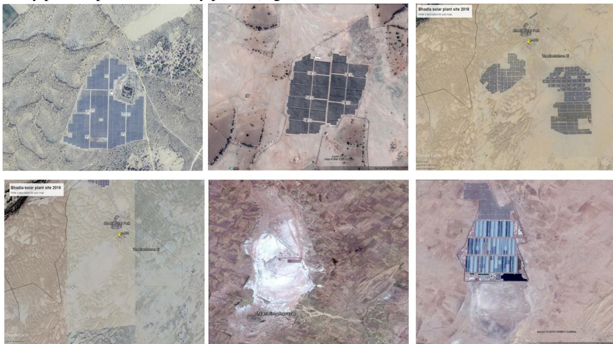
Fig. 4. Solar plant sites on different landforms
