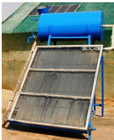
Fig. 5. Natural circulation type solar water heater
