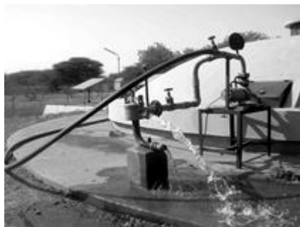
Fig. 3. Operation of pump and blower by PV generator
