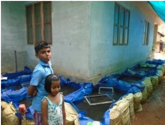
Mud filled cement bag supported pools
