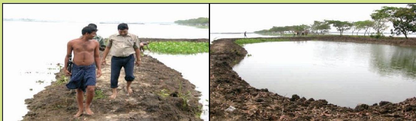
Creation of earthen embankment in waterlogged areas for harvesting floodwater.
