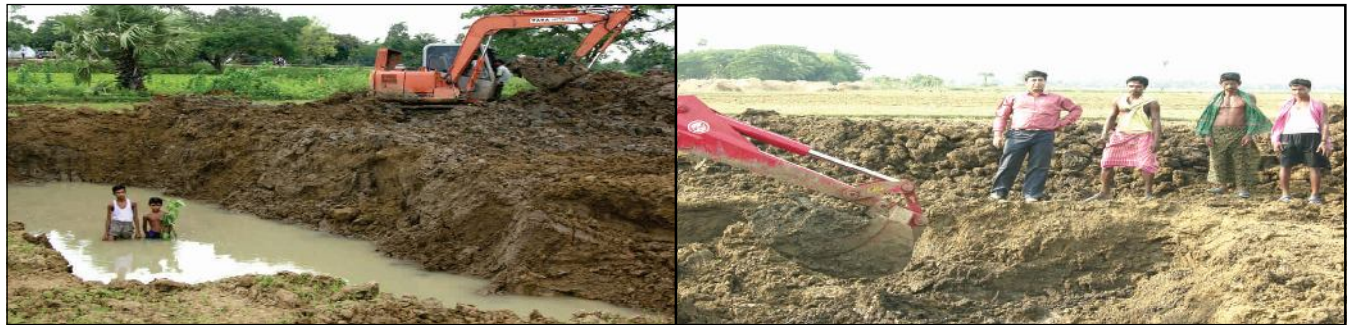
Construction of water harvesting structures is in progress at Sukal, Puri
