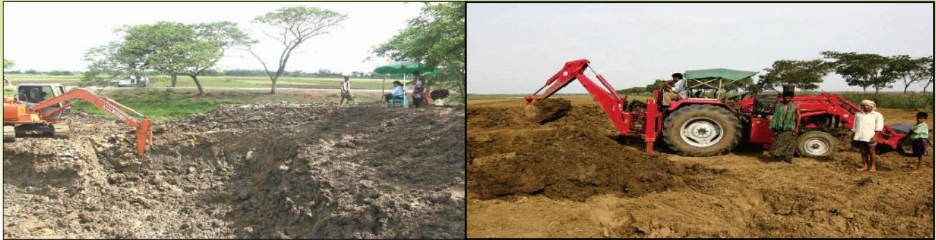
Construction of water harvesting structures is in progress at Alisha, Puri
