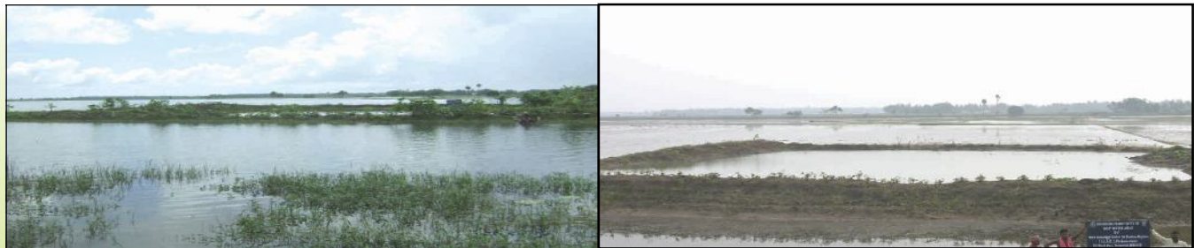
Harvested water inside constructed water harvesting structures during flooding period (August)
