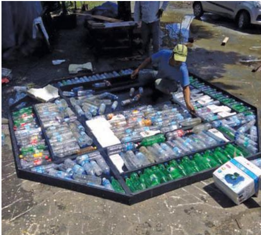
Attachment of recycled plastic bottles beneath the deck
