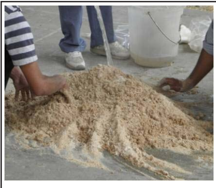
a. Preparation of substrate
