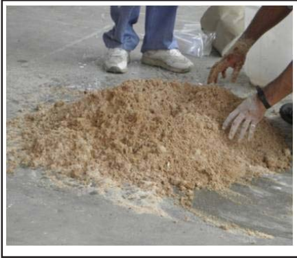
a. Preparation of substrate
