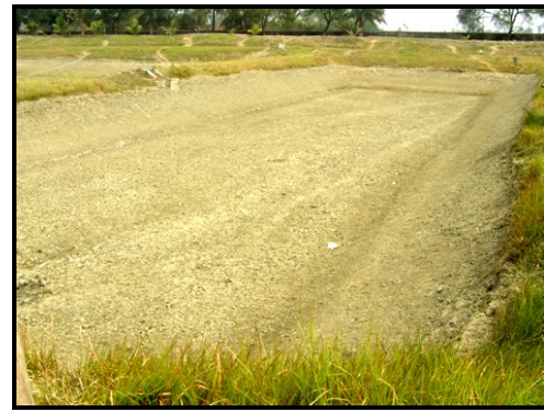
Pond bottom after top soil removal
