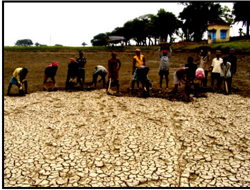
Top soil removal
