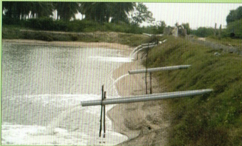
Intake of treated water into grow out ponds
