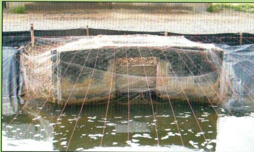
Fencing near sluice gate
