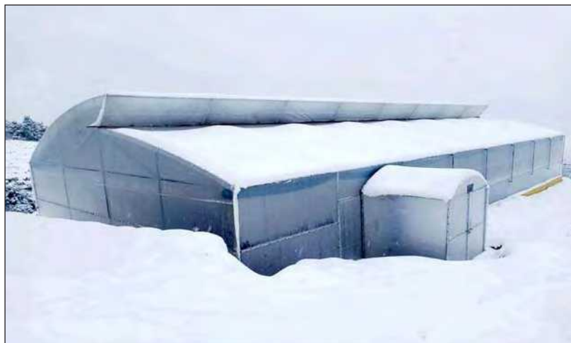
Newly constructed polyhouse (200 m 2 )
