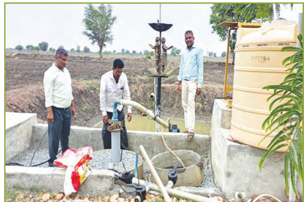
Groundwater point recharge (in progress) during 12 to 14 th May 2023
