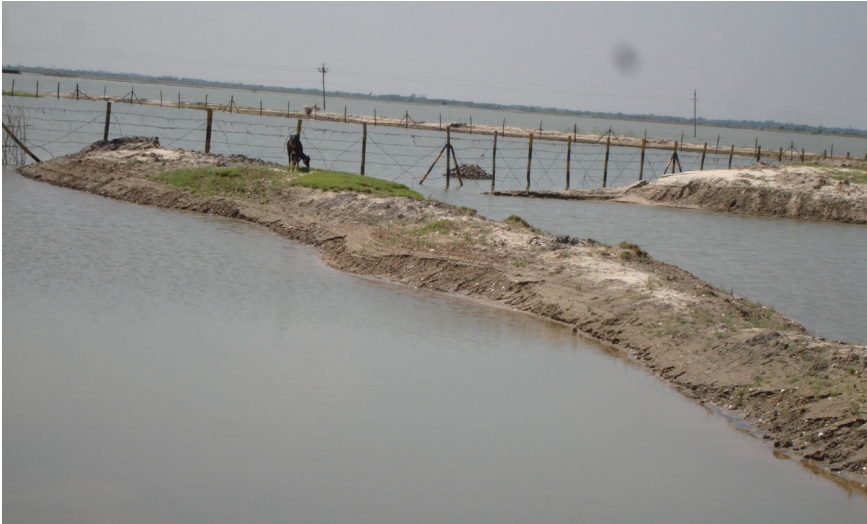
Fig. 8.10. Breaching and inundation of shrimp ponds
