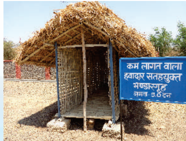
Low volume low cost onion storage structure
