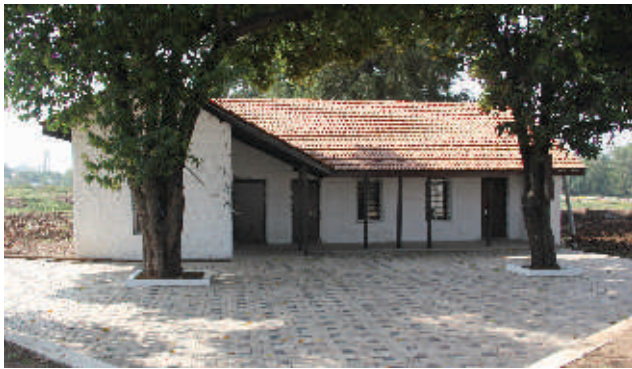
Renovated transit office at Hadapsar Farm
