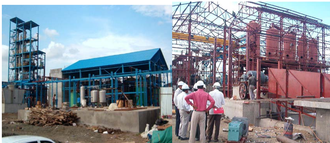
Image.3. 30 KLPD, 900 TCD; 4 tandem mills -sweet sorghum based plant set by M/s Tata chemicals Ltd, Nanded, processing of sweet sorghum for bioethanol. Sweet sorghum is grown over 7000 acres in 2008 and 2009.
