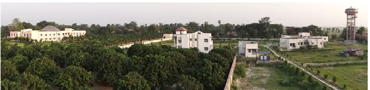
Aerial view of infrastructural facilities created at the centre
