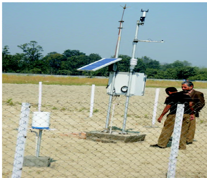
Director, NRCL observing progress of installation of weather station
