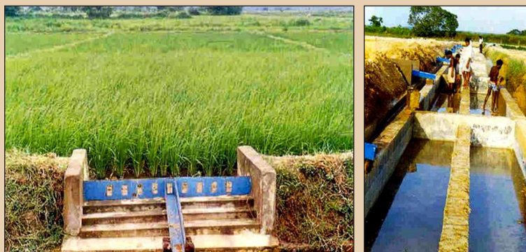
Optimum dike height in rice fields for in-situ conservation of rainwater
