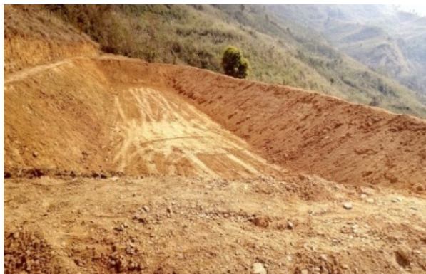
Fig.5 Digging of artificial pond.
