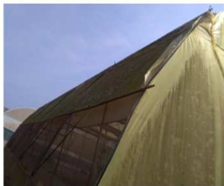
Figure 1. Vertical sides show less algae growth as compared to aerodynamic shape and thus less loss in light transmissivity
