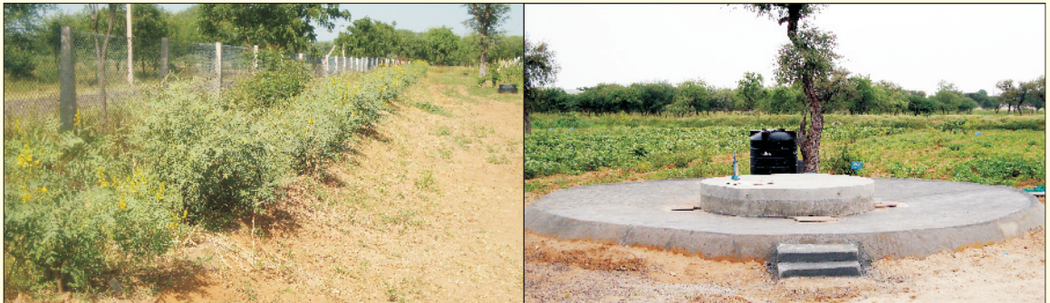
Fig. 23. Field level rainwater harvesting with bunding and ponding.
