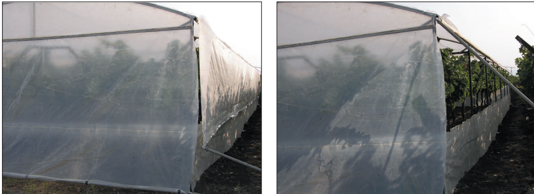
Side view of the plastic structure with side plastic sheet rolled down (a) and rolled up (b)
