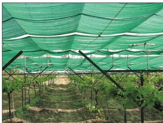
Side view of the plastic structure with side plastic sheet rolled down (a) and rolled up (b)
