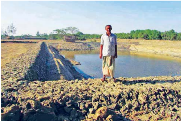
Brackishwater pond excavated at Gangadharpur village
