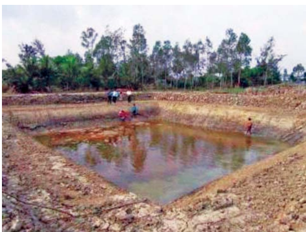
Water harvesting pond of land shaping unit at Uttarchandanpiri village
