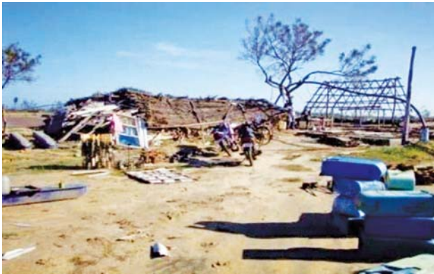
Infrastructure damage to shrimp farms - Uppalavadai
