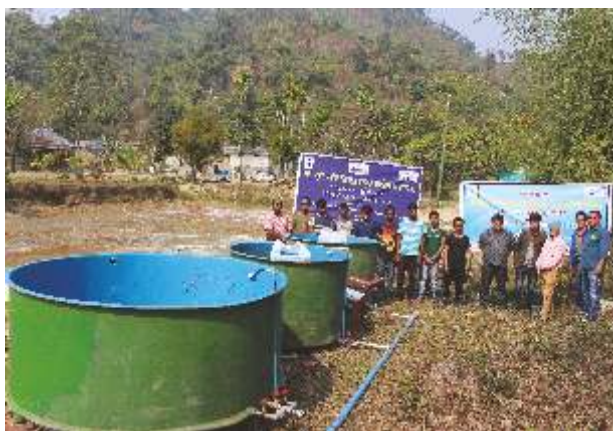
Demonstration of FRP hatchery installation.
