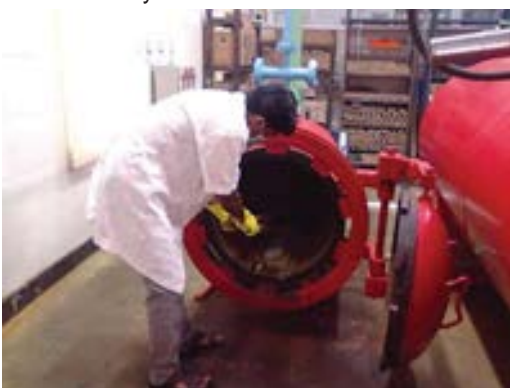
Pilot level wood preservation facility
