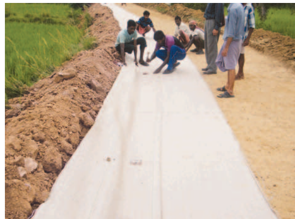
Fig 6 : Anchoring of geotextiles with base soil
