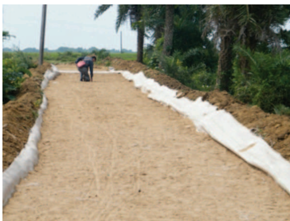
Fig 7 : After spreading of 10 mm thick sand
