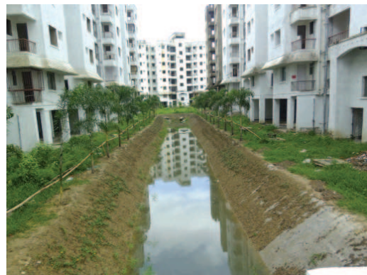
Fig 3 : Condition of trench two months after construction
