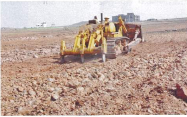
Ripping and chaining with heavy machineries
