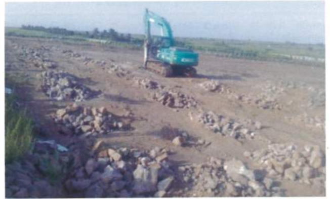
Making pits using hole diggers
