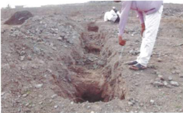
Trench after blasting below planing sites
