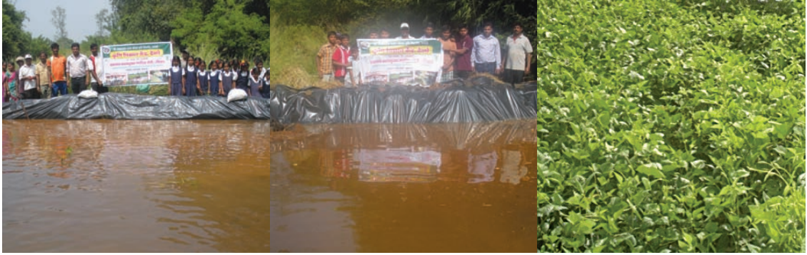
Construction of Konkan Vijay Bhandaras for rain water harvesting
