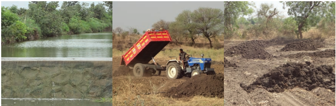
Renovated Check Dam
