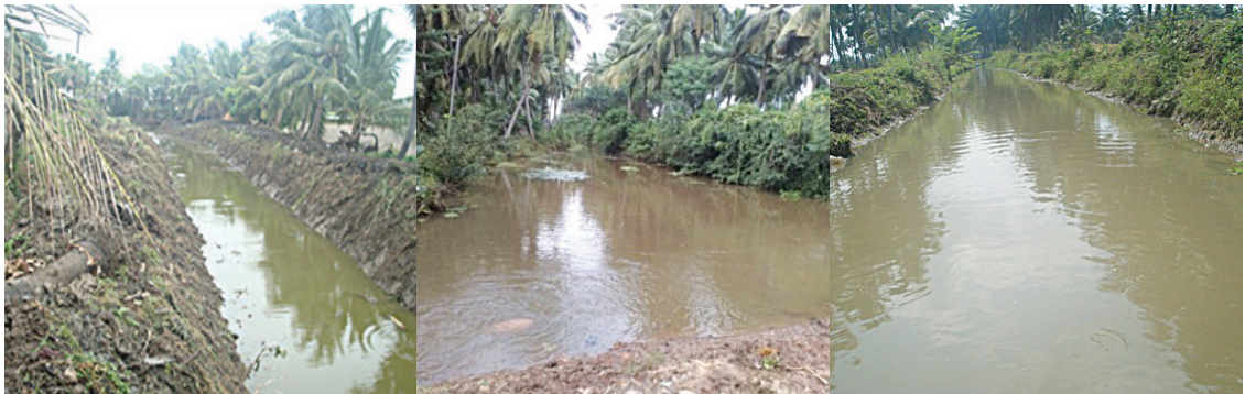
Renovation of Matsyapuri drainage channel
