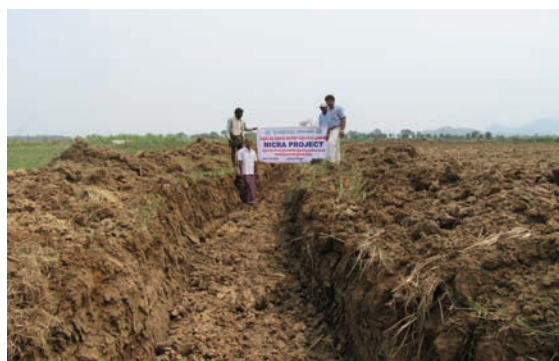
Field drainage channel
