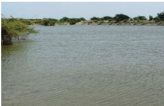
Percolation tank after desilting
