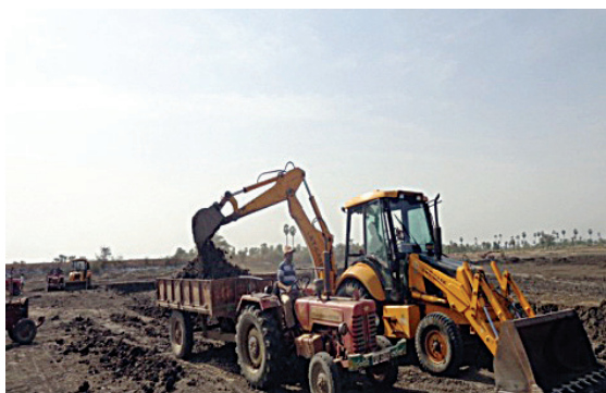
Desilting of village tank
