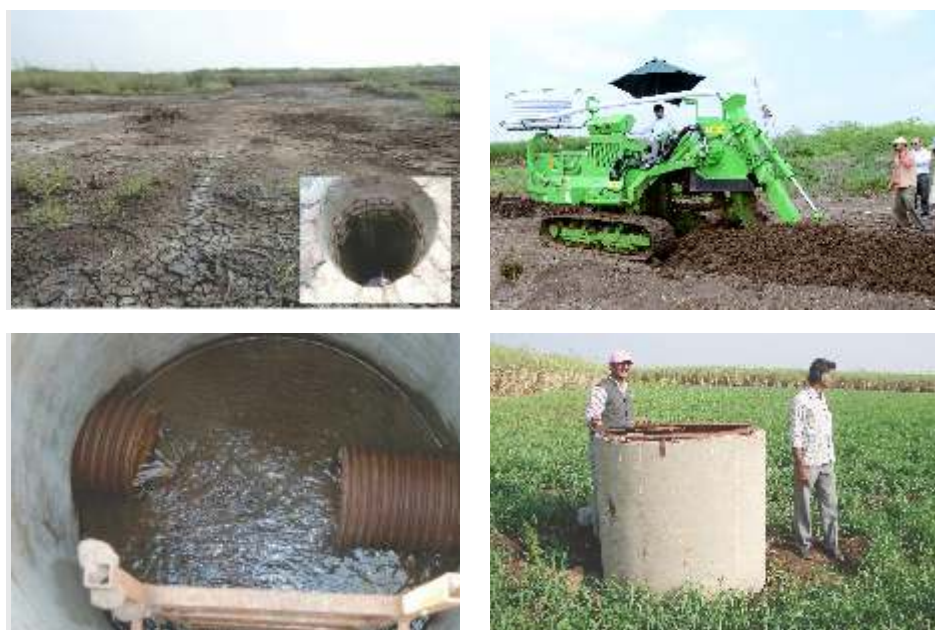
Fig 2.2. Pre-project field condition, installation of SSD system and saline water flow in collectors to open drain (top row); and good crops after SSD installation (bottom row)
