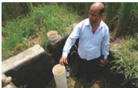
Fig 6.4. Groundwater recharge structure
