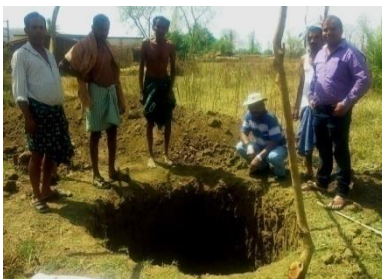
Digging of open well
