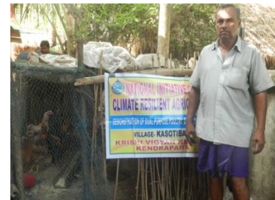
Low cost brick structure for poultry shed
