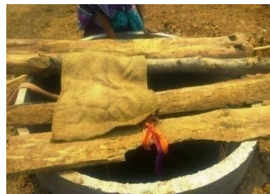
Fully constructed open well
