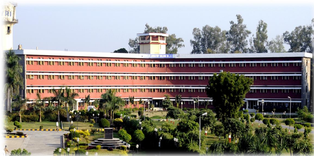
Modular Laboratory Building, ICAR-IVRI, Izatnagar, Bareilly (U.P.), India
