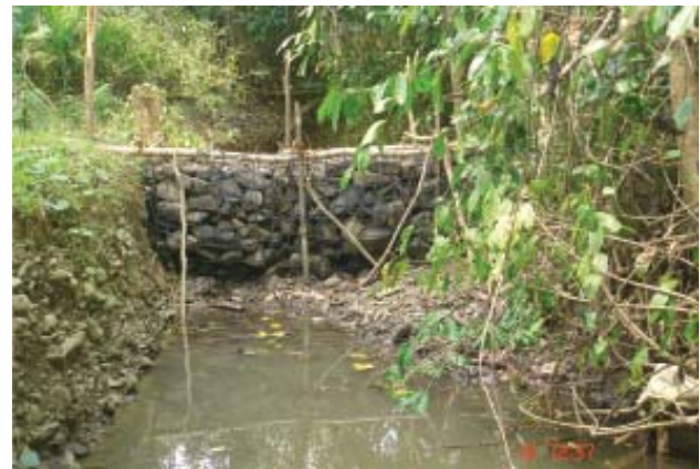
Fig.10. Gabions constructed through water user association in Manjeri village
