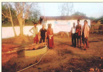
Ring well construction
