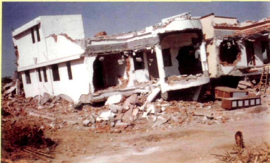
Badly damaged building in Lakadiya village
