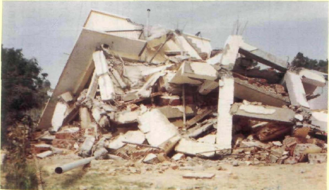
Plate 6. Collapsed PHED building near Manfara village
