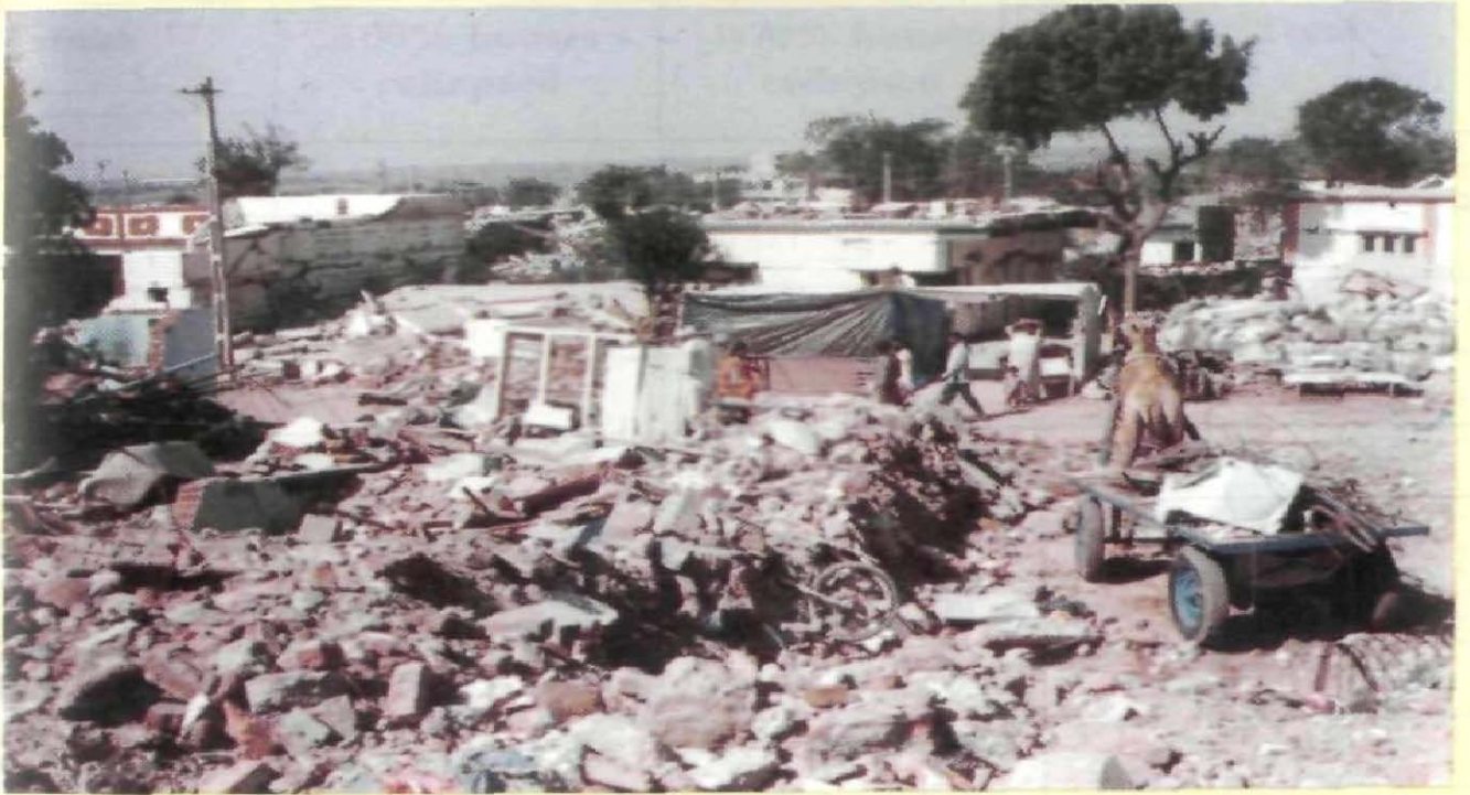
Plate 7. A scene of very severely affected Bhachau town
