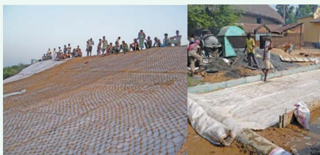
Riverbank protection by geotextile Rural road construction by geotextile
