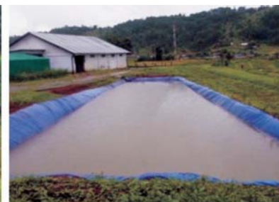
Micro-rainwater-harvesting structure ( Jalkund )
