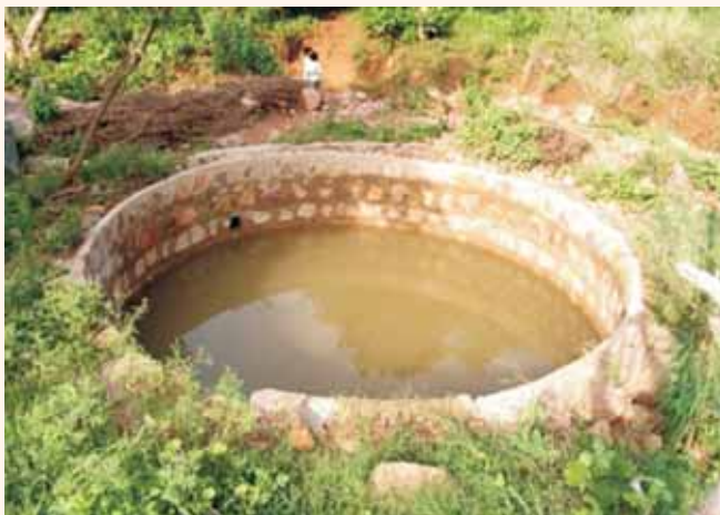
Recharge in wells of Garhkundar Watershed
