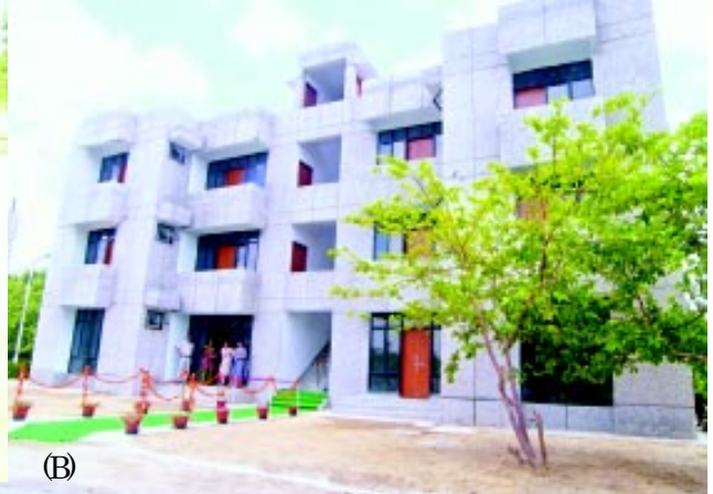
Fig. 62. The newly constructed residential block (B)
