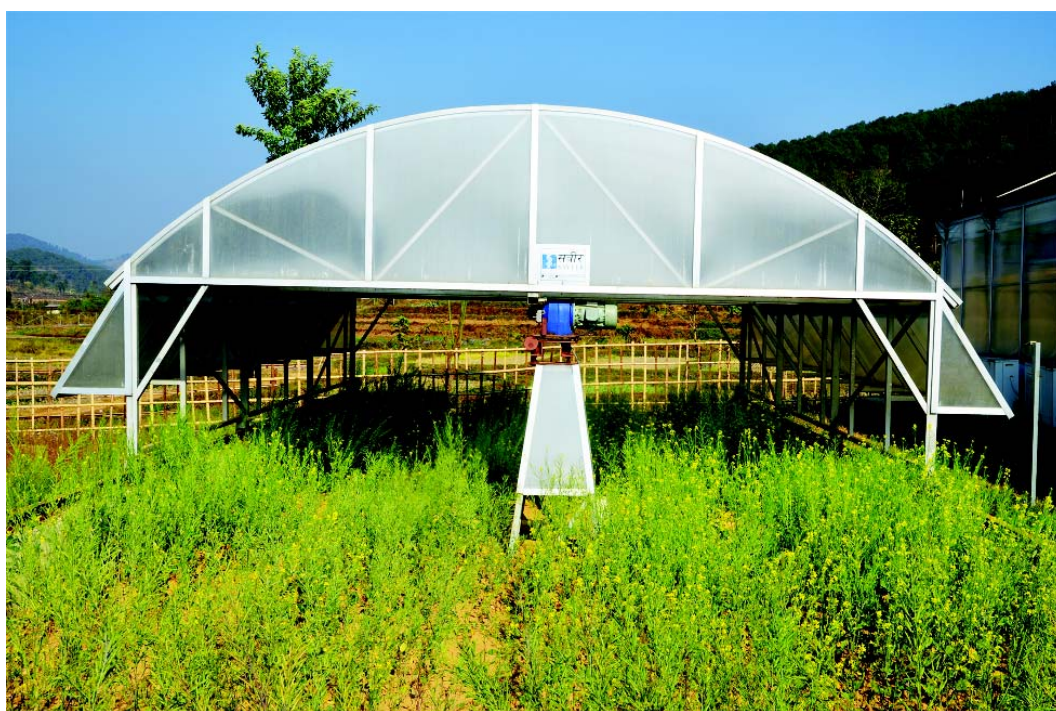
Automatic rain out shelter facility at ICAR RC NEH Region
