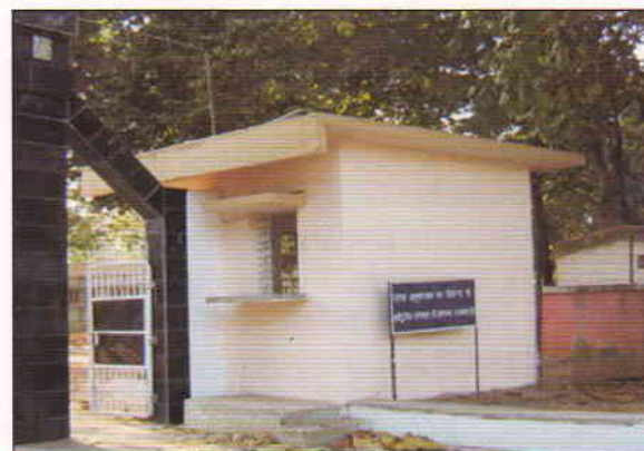
Fig. 48b. Security Post painted with shellac emulsion paint
