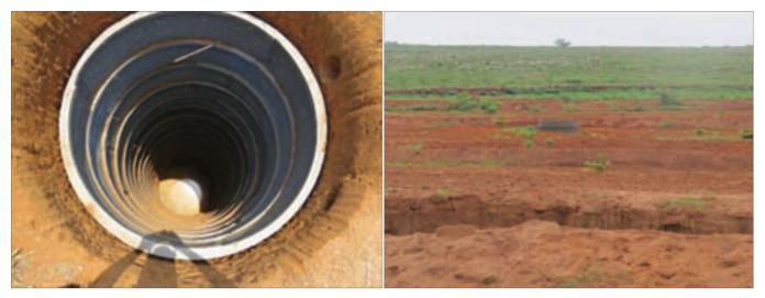
Open well in the terraced field getting recharged at higher rate due to increased runoff retention in the terraced portion and thus allowing more ground water recharge
