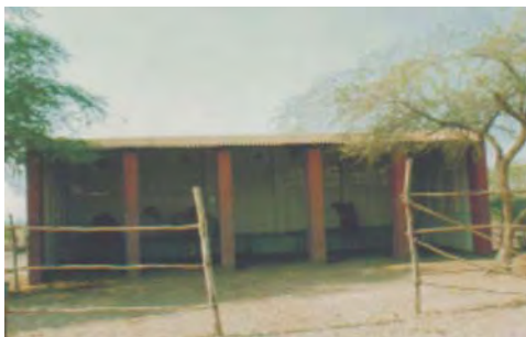
Shed with asbestos roof
