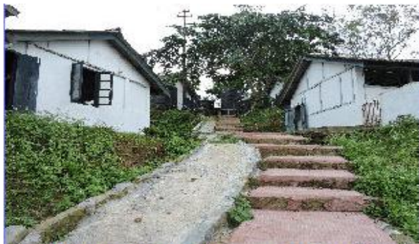
Internal footh-path re-constructed during 2014-2015
