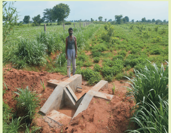
Haveli renovation in Parasai-Sindh watershed; Masonry drop spillway (rectangular weir) and embankment along with corewall was constructed in 50 m breached area. Water harvested in Haveli during the monsoon period.
